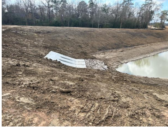
February 7, 2025 Constructed Detention Pond Outfall
