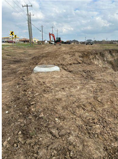
February 5, 2025 New Manhole Installation
