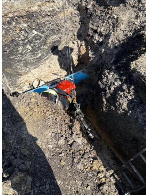
February 7, 2025 TS&V Installation at SH-105
