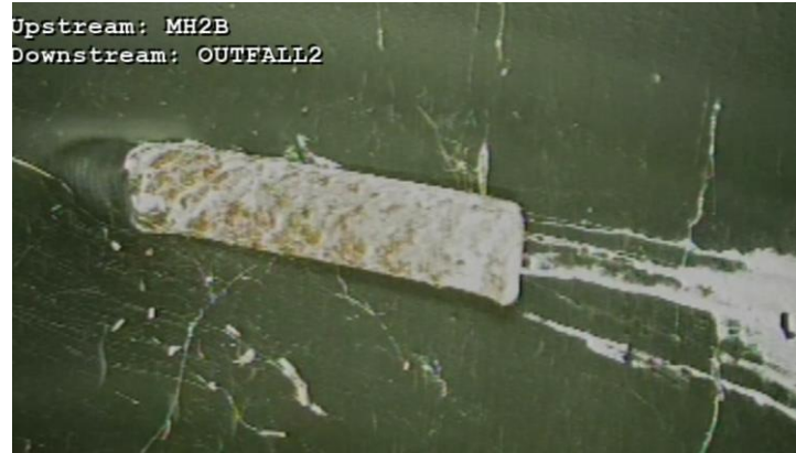
Figure 2: Rebar Penetration
