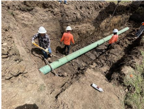
Figure 1: Installation of offsite waterline April 11 th
