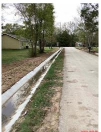
Figure 1: Newly Constructed Roadside Ditch along McGinnis November 15, 2022
