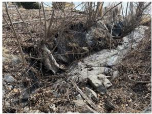
Figure 2. Erosion in the channel (looking south, Lake Minnetonka in the background)
