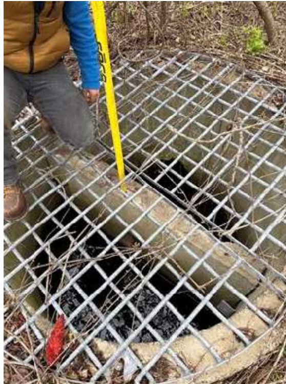
Figure 10: Outlet Control Structure (NW)
