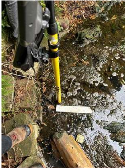
Figure 13: 12" RCP Outlet (S)
