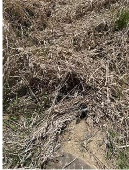
Figure 2: 12" RCP Outlet (NE)
