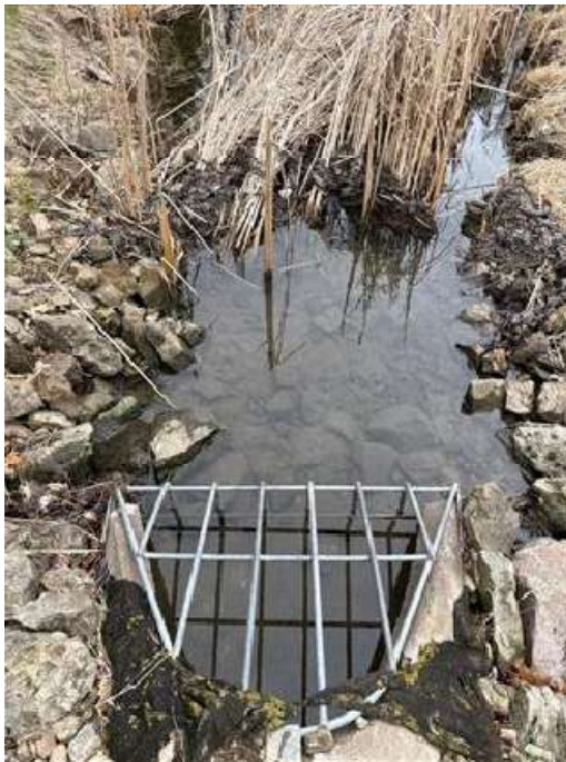
Figure 3: 18" RCP Inlet (N)
