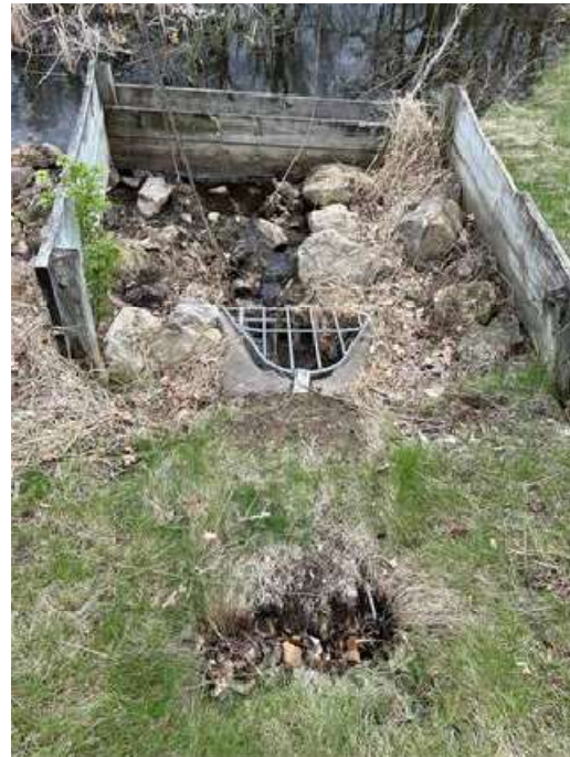
Figure 4: 15" RCP Outlet (W)
