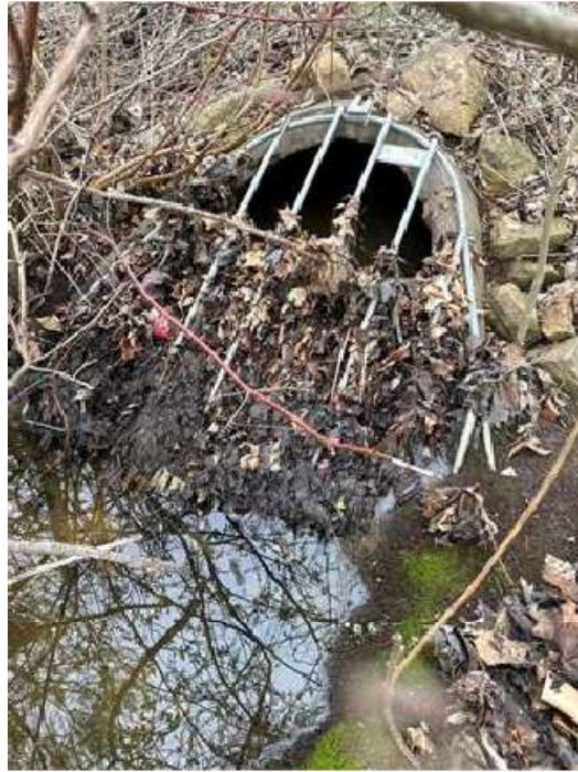
Figure 7: 24" RCP Inlet (N)
