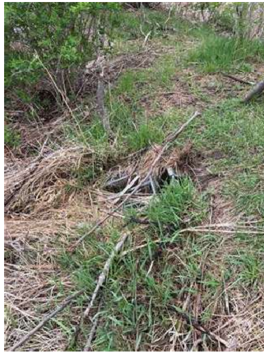
Figure 15: 12" RCP Outlet (E)
