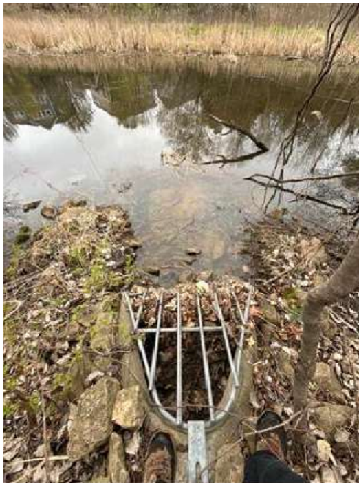
Figure 5: 15" RCP Inlet (SW)
