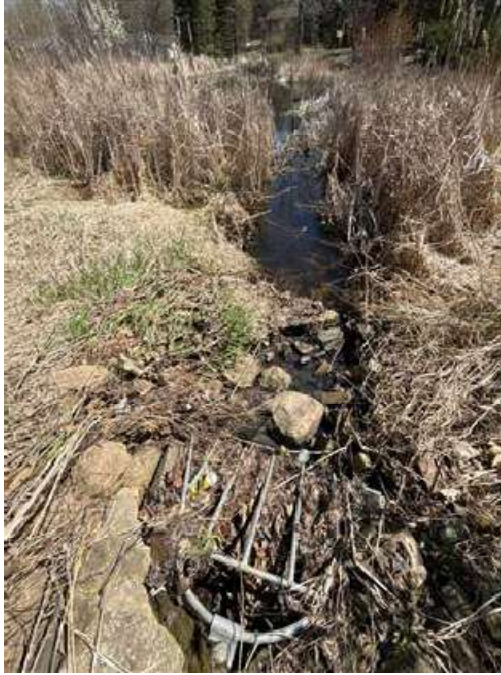
Figure 1: 18" RCP Inlet (SW)
