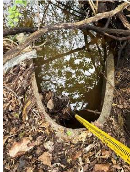
Figure 12: 15" RCP Inlet (SW)
