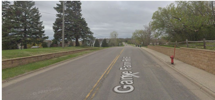
Figure 1. Hydrant along Game Farm Road, west of CR 110
