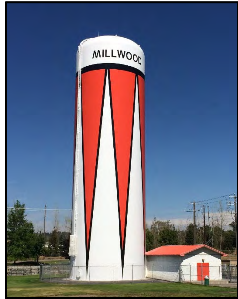
Figure 11-2: Millwood Water Tower
