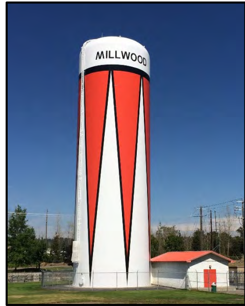
Figure 11- 12 : Millwood Water Tower
