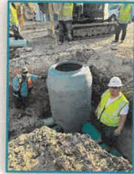
Dunlap / 1 st - Replaced Manhole
