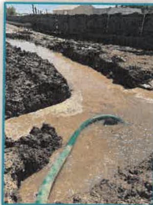
Conway / Military Repair of Water Break
