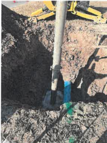
28 th /Conway Sewer Line Repair
