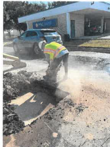
Conway/Bus 83 Water Line Repair
