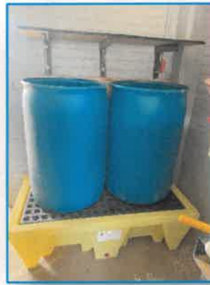
Chemical Day Tanks & Spill Protector -SWTP
