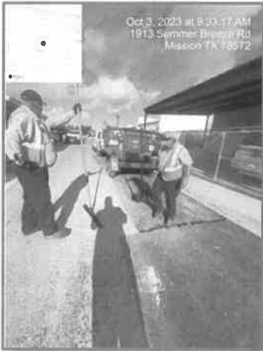
Summer Breeze Road Maintenance
