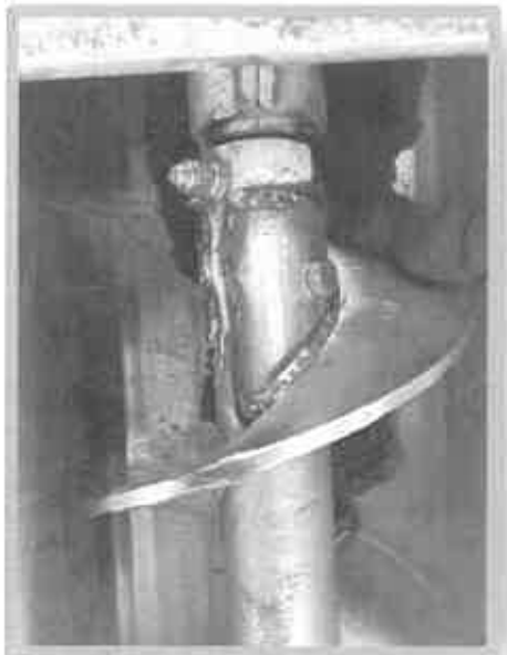
Maintenance to Auger
