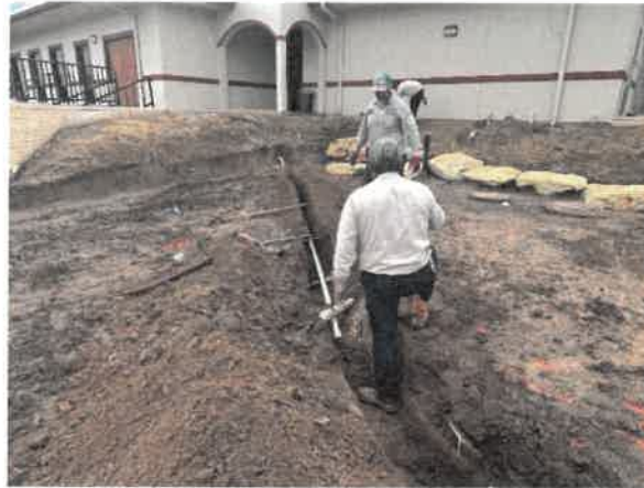
Placement of Retaining wall with boulders from Bannworth Park Pond / Irrigation Mainline Installation
