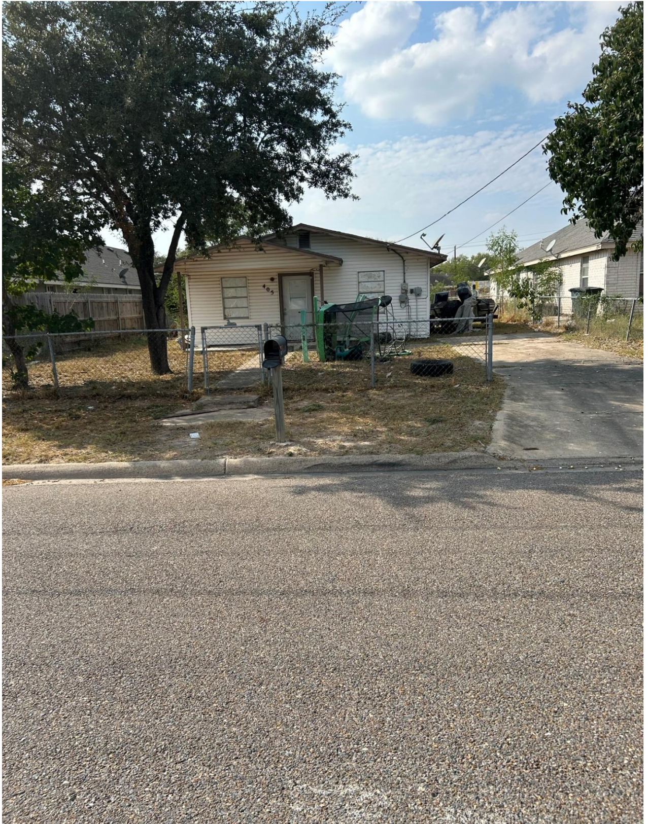
PHOTO OF THE SUBJECT PROPERTY
