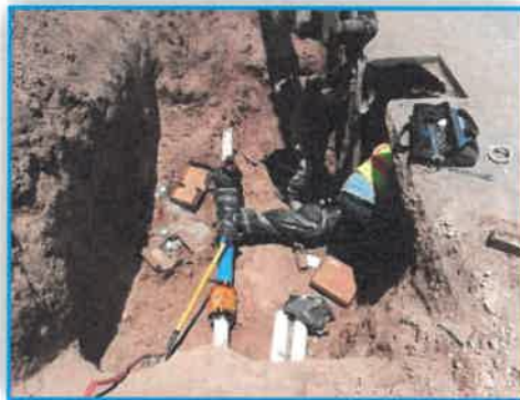
Amber Grove - 8 Inch Water Line Connection
