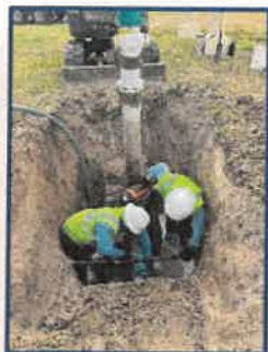
201 Melba Carter Hydrant T-Line Break Repair
