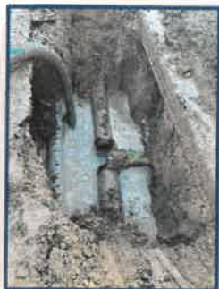
201 Melba Carter Hydrant T-Line Break Repair
