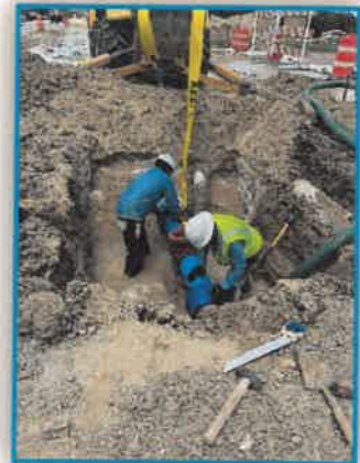
Los Ebanos / Mile 1 South Repair of Water Break
