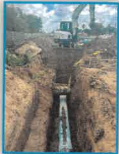
Conway / Los Indios Repair of Water Break
