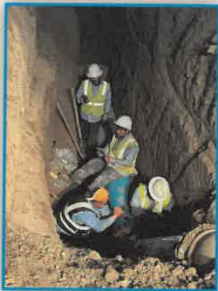
Conway / Los Indios Repair of Water Break
