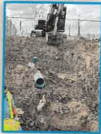
1300 S. Conway – Repair of 10-Inch Sewer Line
