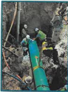
La Lomita / Del Mar Sewer Line Repair
