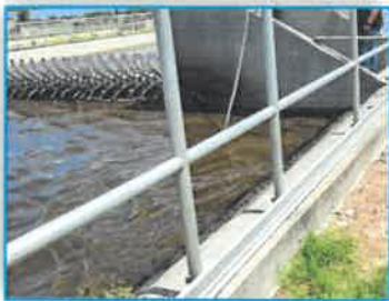
Rotor System Repair
