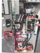
Lift Sta. Pump 6 Maint.
