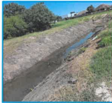
K-Mart Drain Ditch Long Reach Excavator Clean Out
