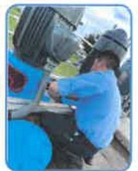
Train C Transfer Pumps Coating NWTP
