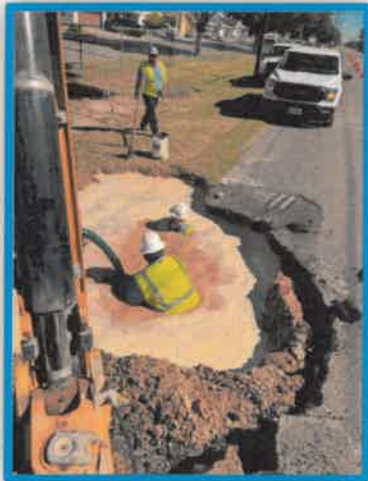
Water Break Repair Stewart / Aladdin Villas
