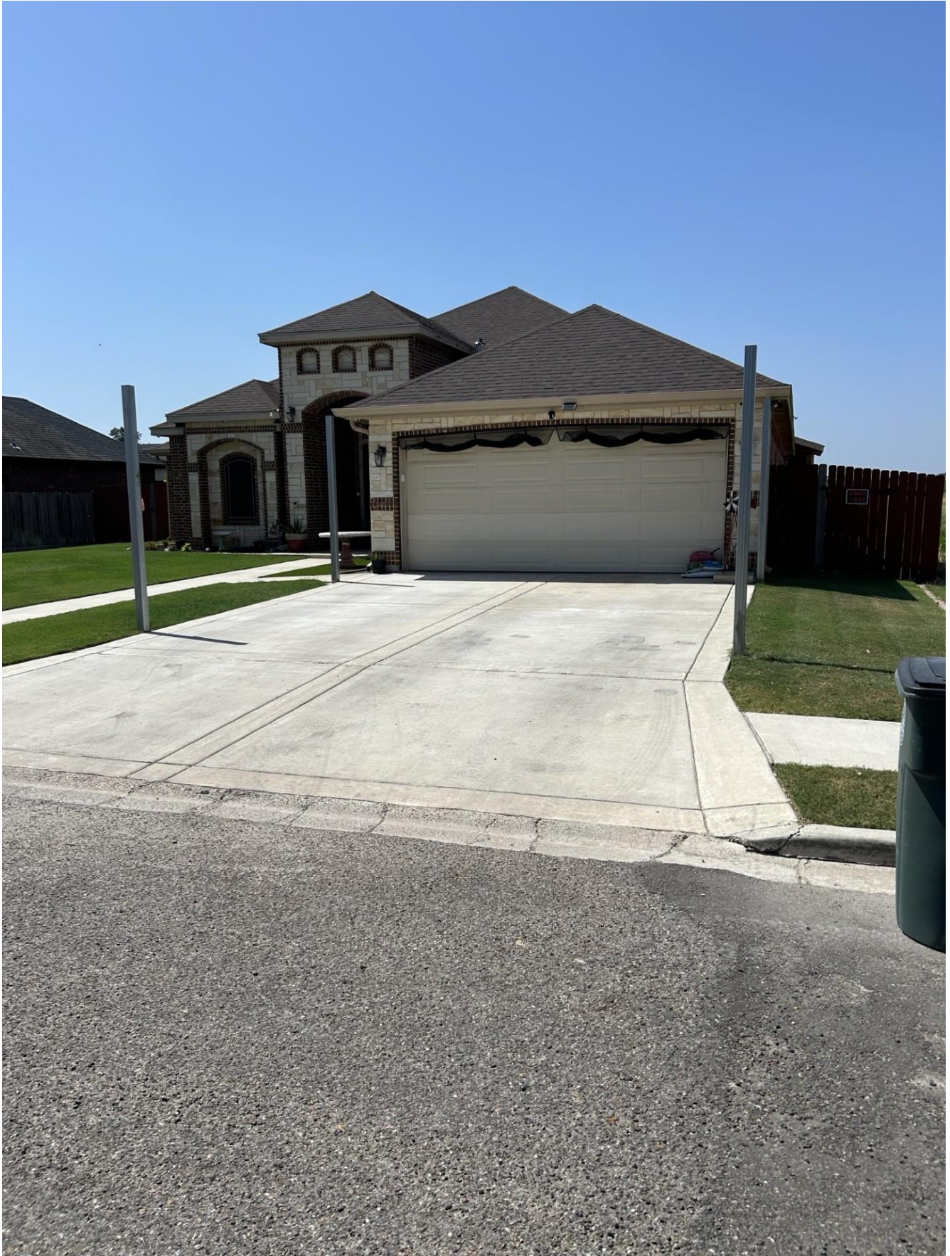
EXISTING HOUSE ALONG LAS BRISAS STREET
