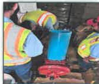
12" Valve Installation
