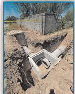
Azalea Storm Drainage Project
