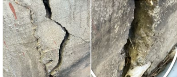
(Detail 9) Cracking Foundation.
