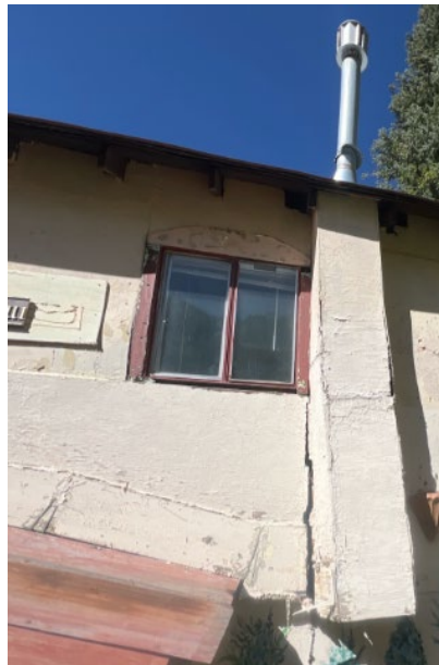
(Detail 10) Deteriorating foam chimney.
