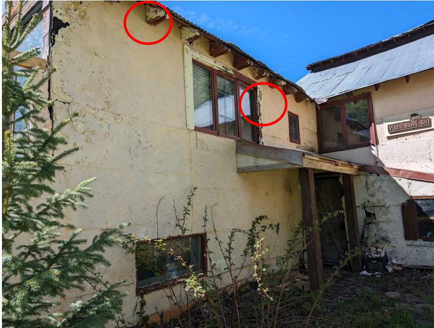
(Detail 1) Foam forms and “siding” on rear addition.
