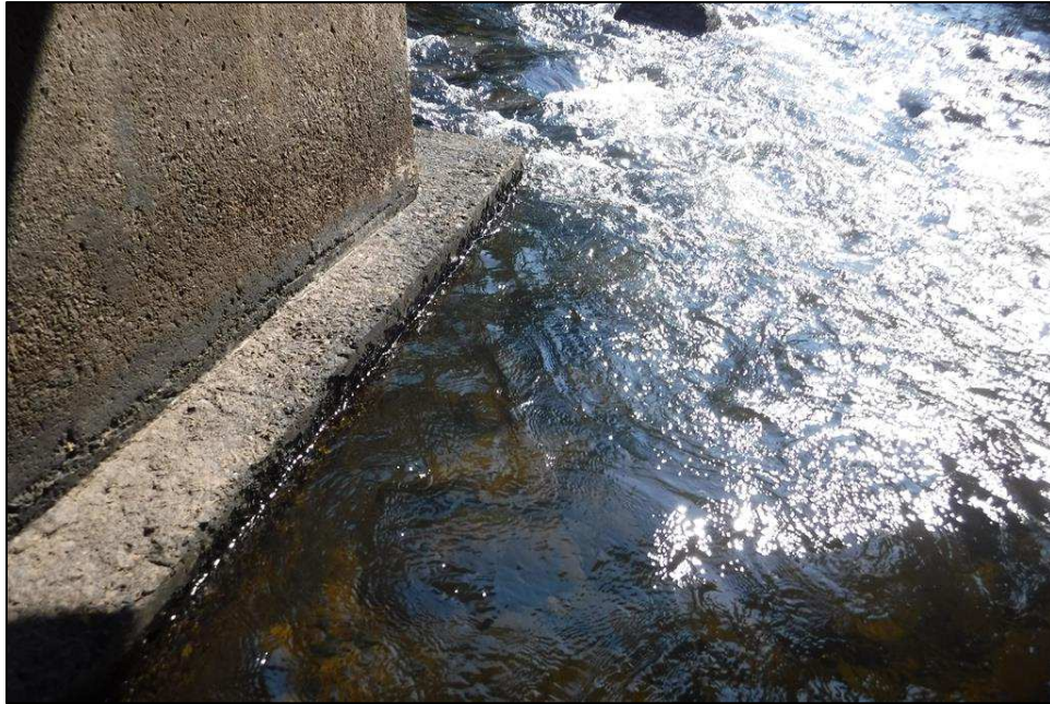
P4 south side exposed footing.
