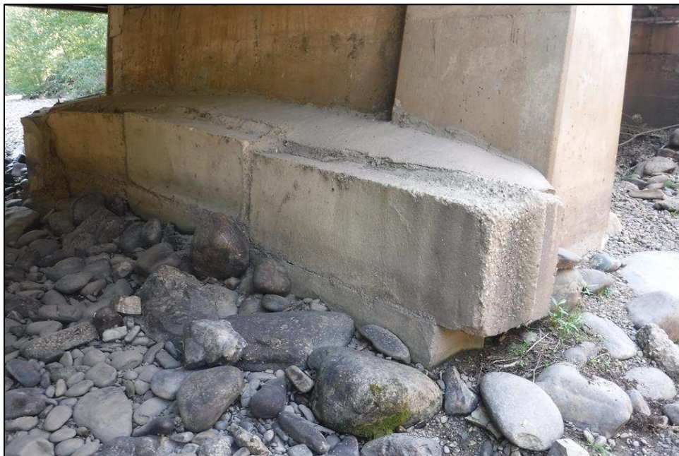
Pier 2 exposed footer.
