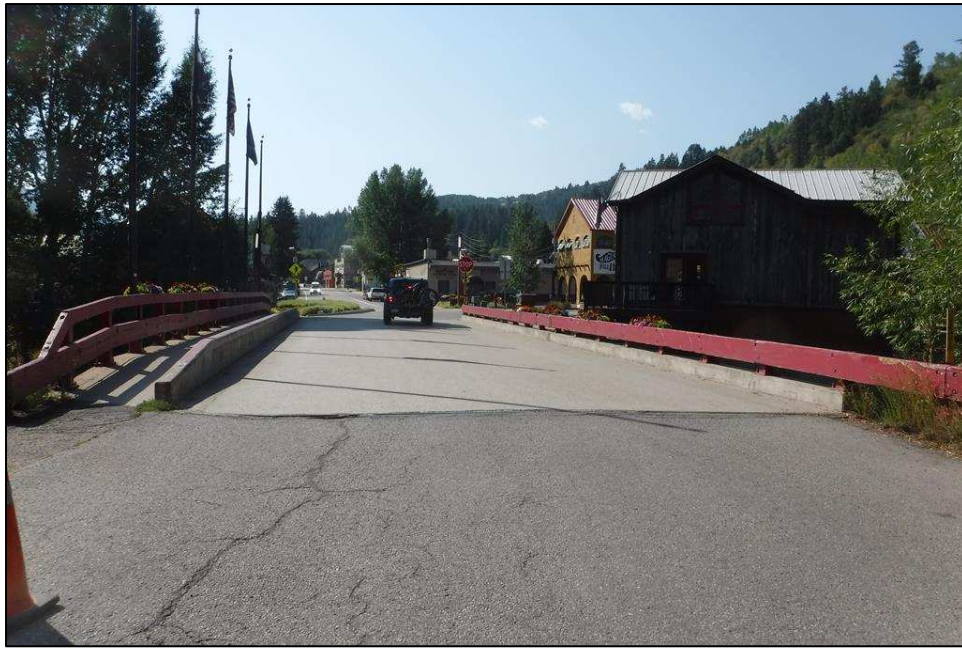
Roadway looking south.
