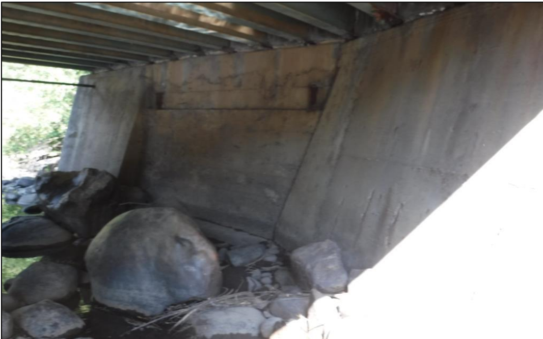
General view of Abutment 5.
