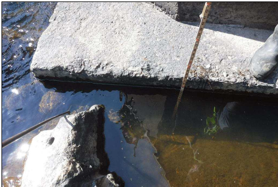
P4 northwest corner exposed footing.
