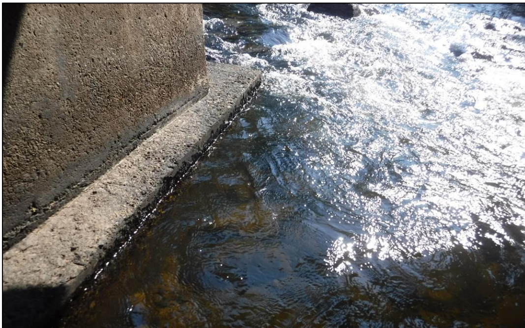
P4 exposed footing at south side.
