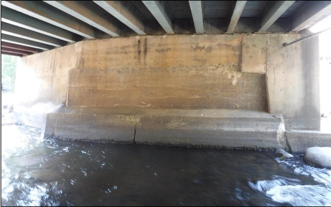
General view of Pier 3.
