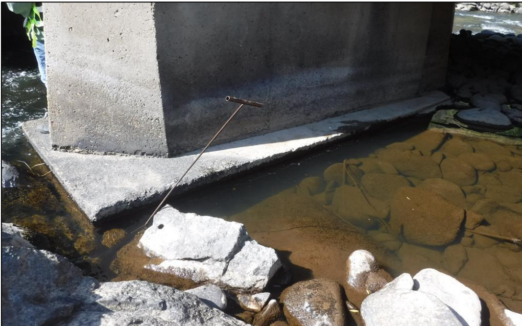
P4 exposed footing at north side.
