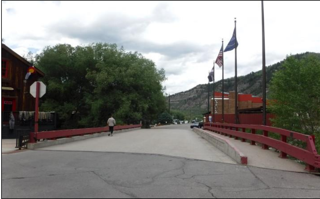
Roadway looking north.
