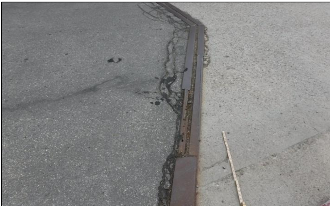
General view of south expansion joint.
