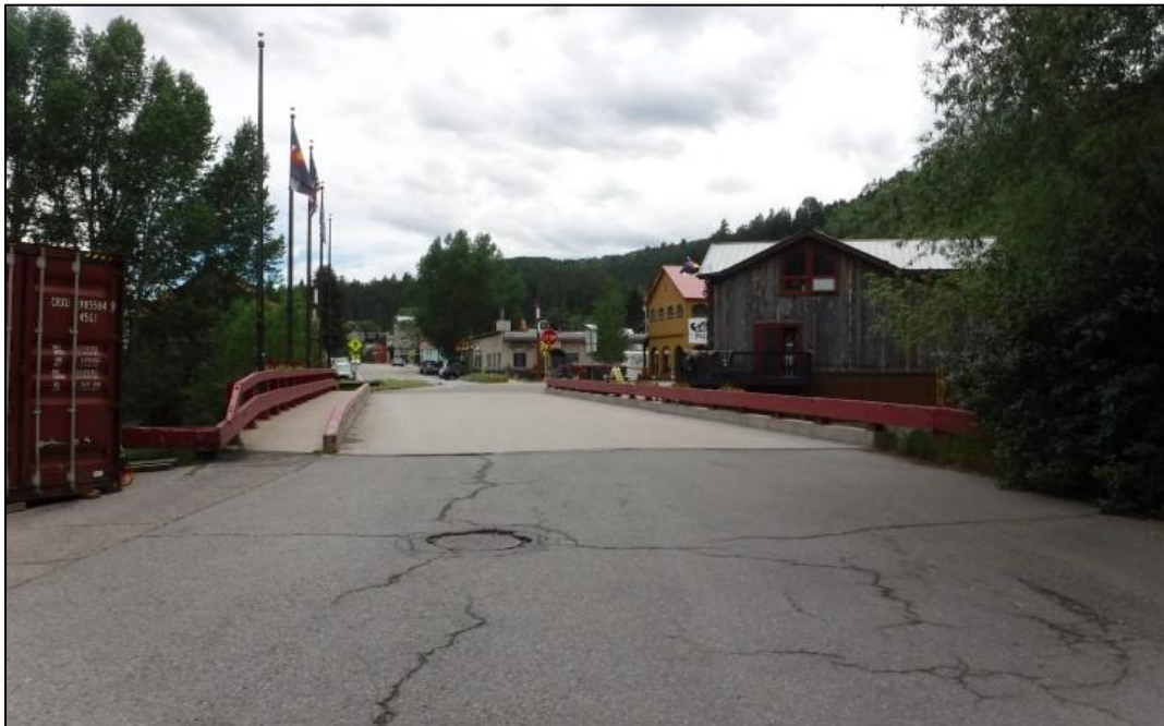
Roadway looking south.
