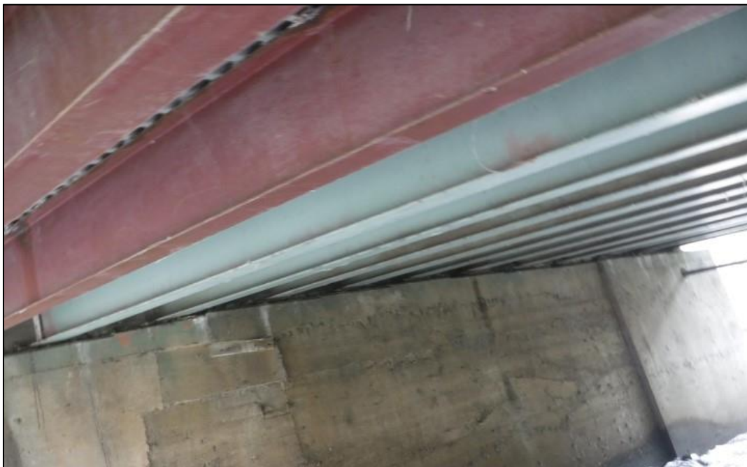
Superstructure looking north.
