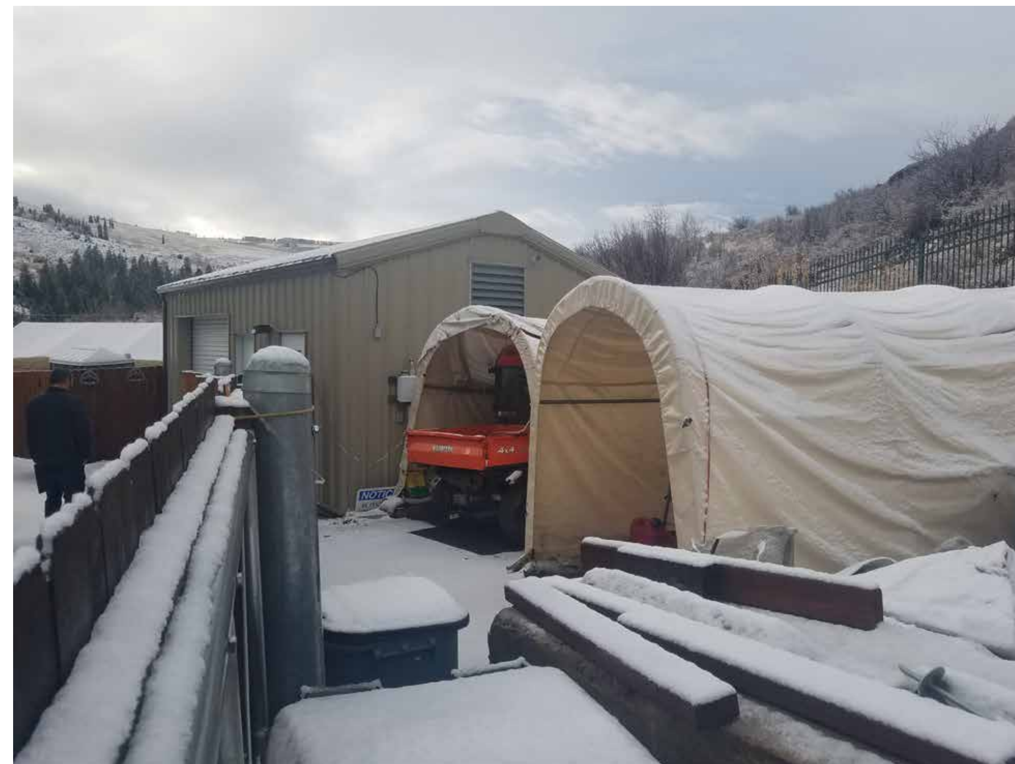
Existing temporary storage
