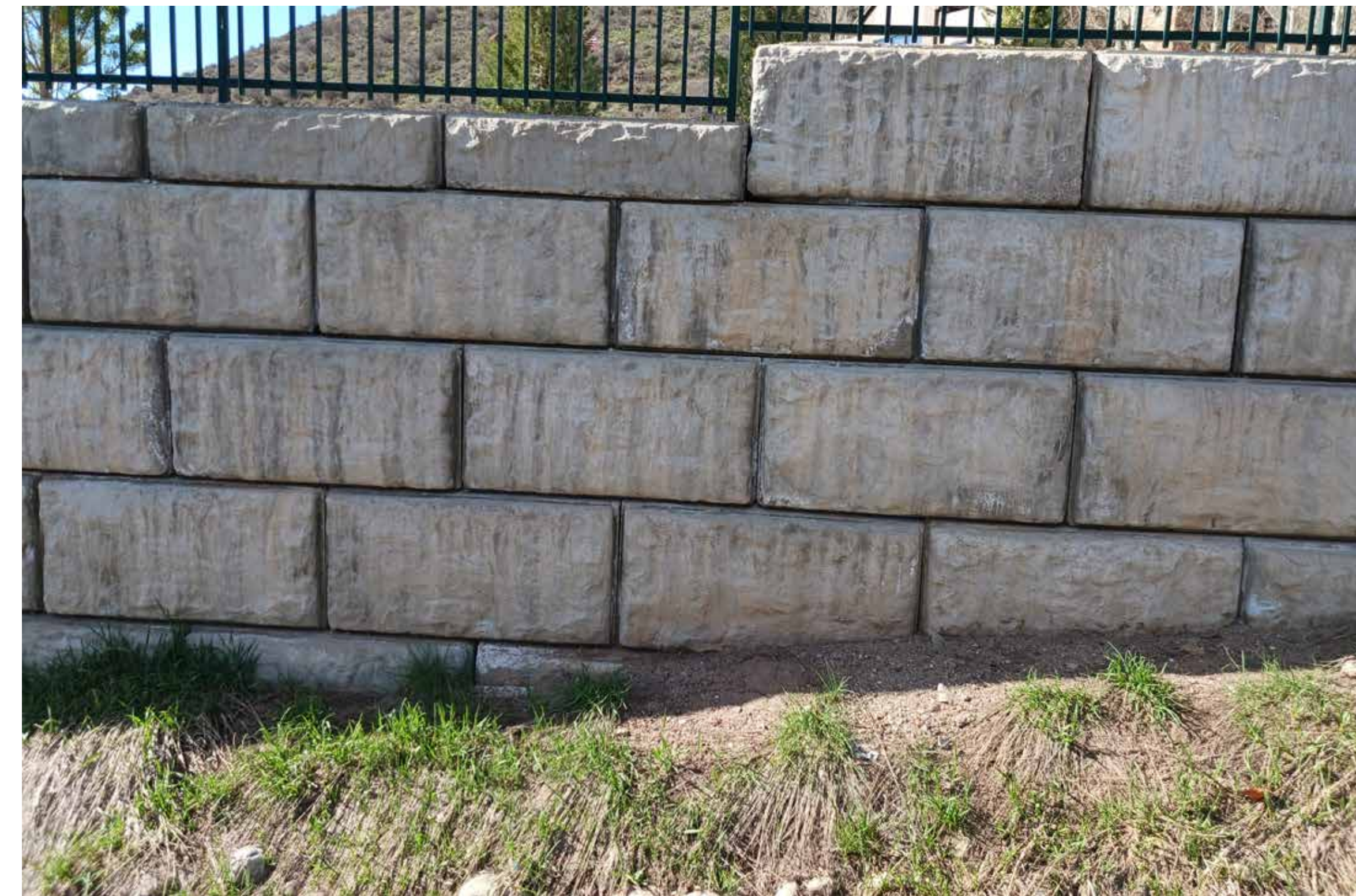
Existing Concrete Block Wall
