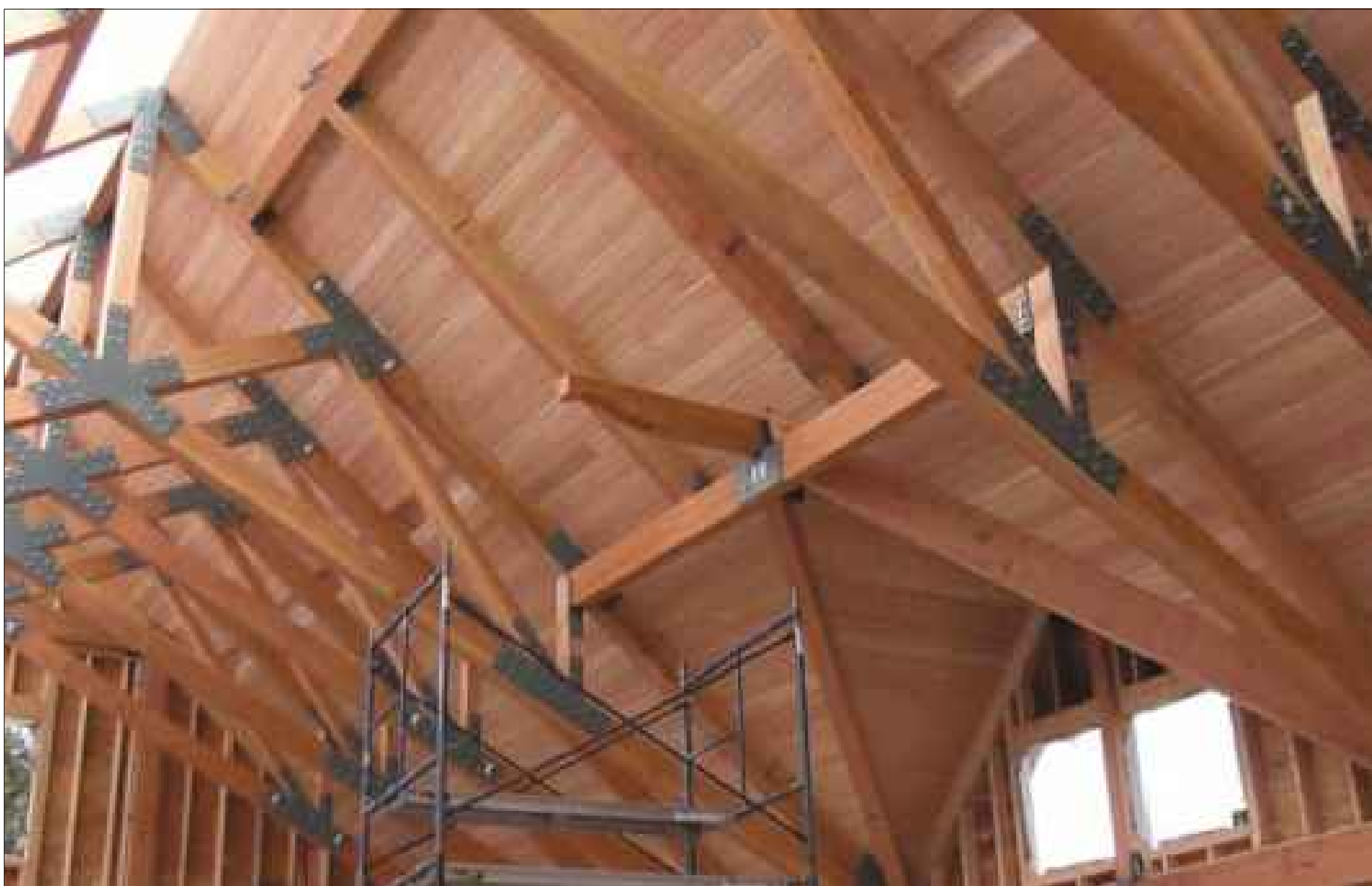
HEAVY TIMBERS WITH STEEL PLATES AND BOLTS
