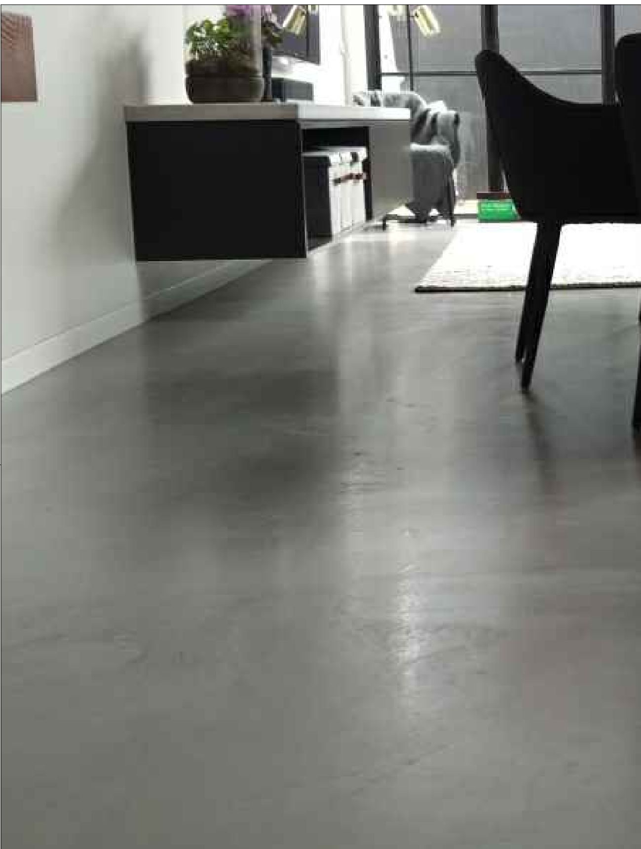
BURNISHED CONCRETE FLOORING. TO BE USED ON ALL FLOORS AS FINISH MATERIAL.
