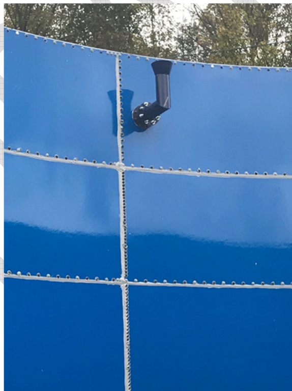
Figure 8: Finished Panel Bolted Tank
