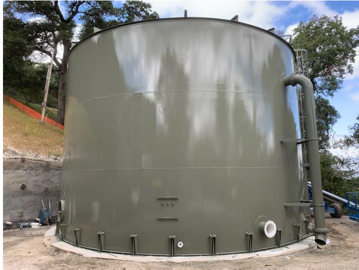
Figure 7: Finished Welded Tank
