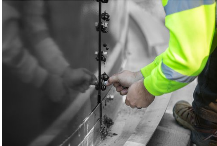
Figure 6: Bolted Tank Blast, Recoat and Reseal
