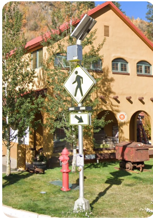
Figure 6: A Rectangular Rapid Flashing Beacon in downtown Minturn from Google Maps Street View
