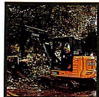
Downed / Hazardous Tree Removal
