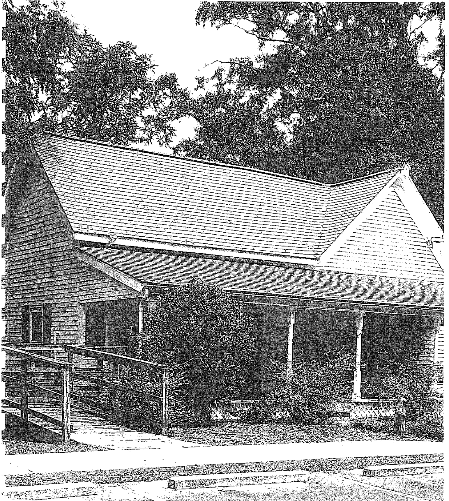
Front of 13560 Cogburn Road – May 2023
