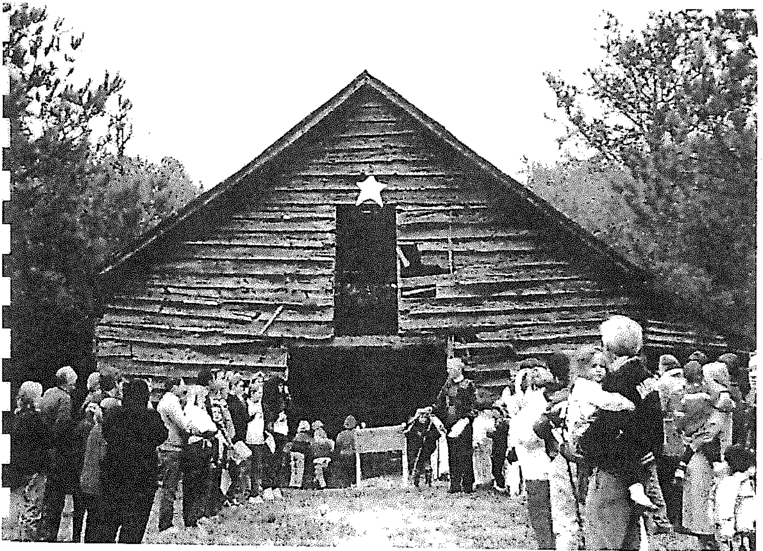
Old Barn at 13560 Cogburn Road
