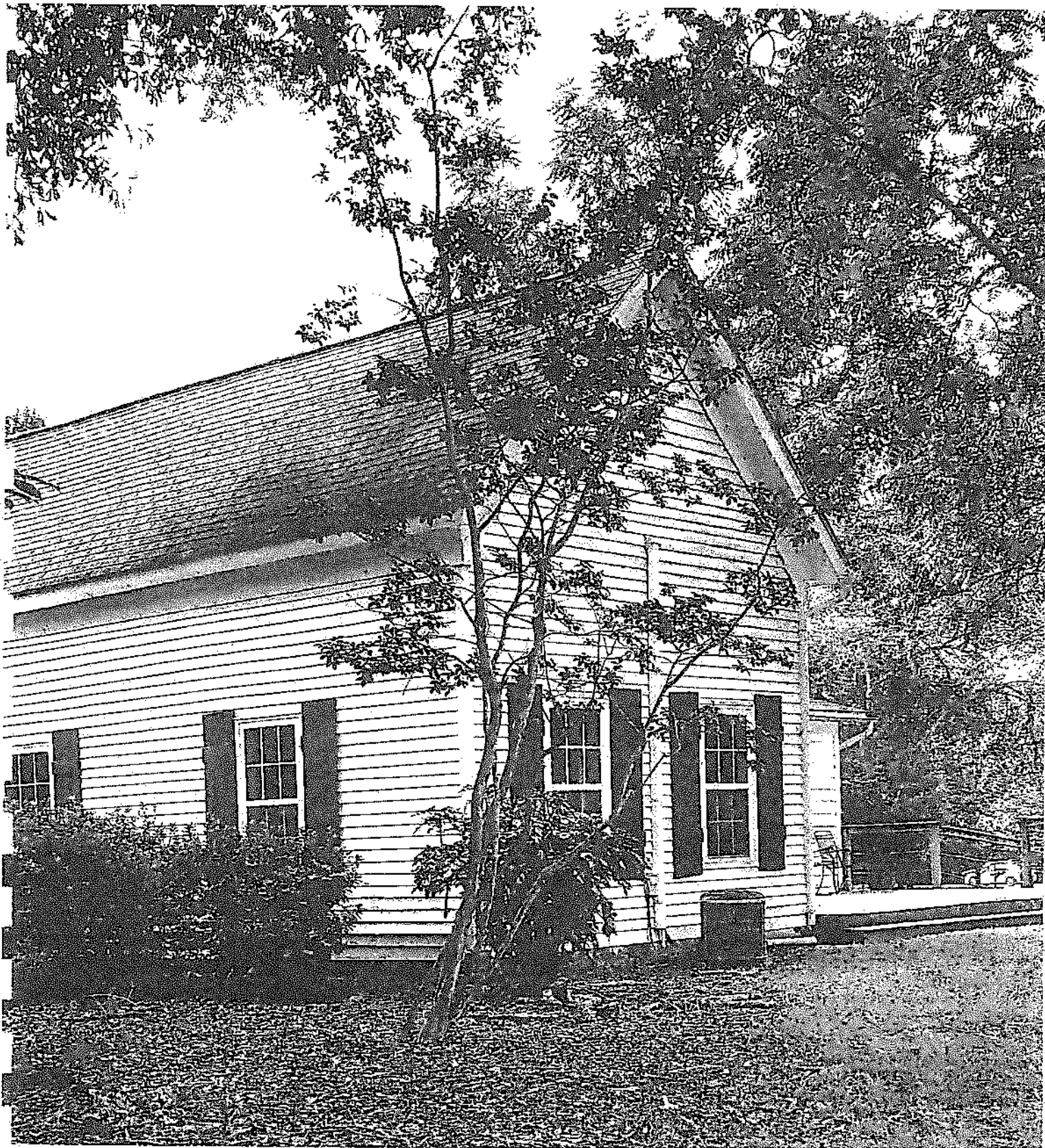
Rear of 13560 Cogburn Road – May 2023
