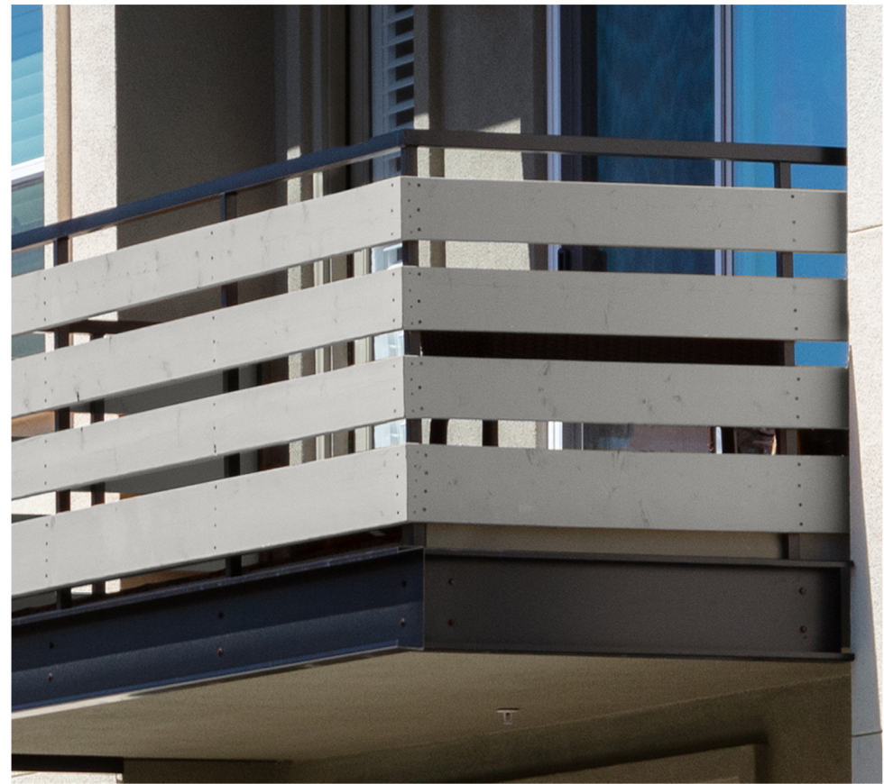
7 METAL RAILING WITH HORIZONTAL WOOD PLANK RAILS
