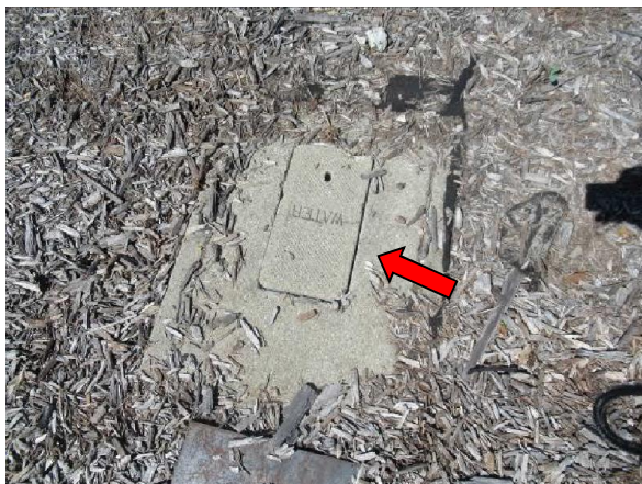
Photo #37 View of the water meter manhole.
