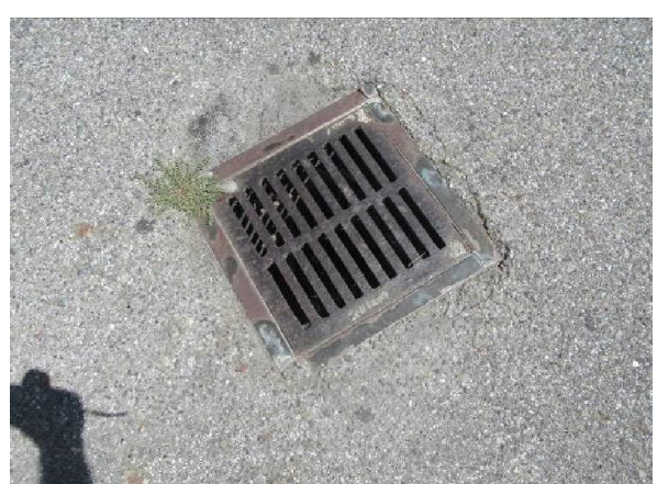
Photo #38 Typical storm water manhole.
