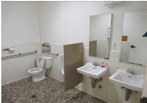
Photo #21 View of plumbing fixtures in the men's restroom.
