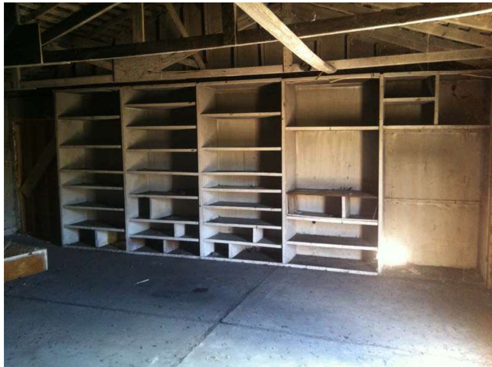
Photo 4: View inside of on-site garage. Photo taken July 2015.
