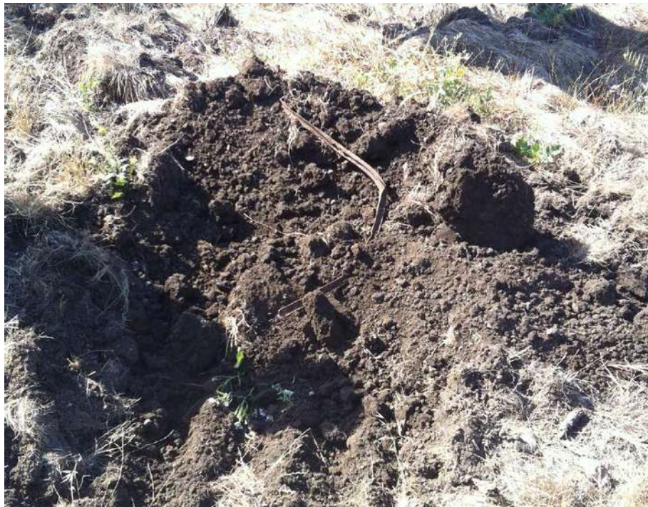
Photo 8: View of typical fence post uncovered during potholing of magnetic anomalies. Photo taken in June 2015.
