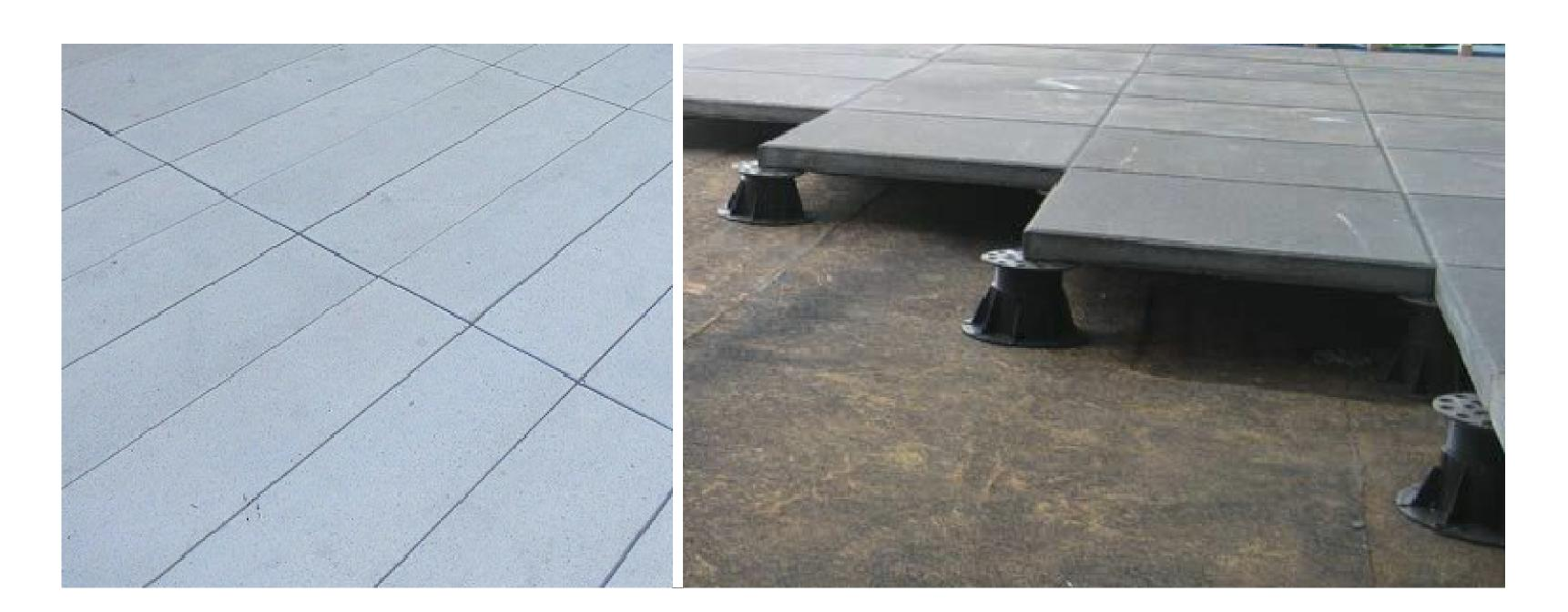
CONCRETE PAVERS ON VERSADJUST PEDESTALS
