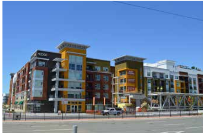
The Edge Apartments: New high-density mixed-use development directly across Montague Expressway from the Milpitas Transit Center.
