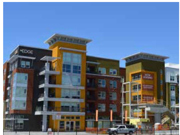
Articulated facades - Architectural features and changes in massing are used to create visual interest on the building facade.
