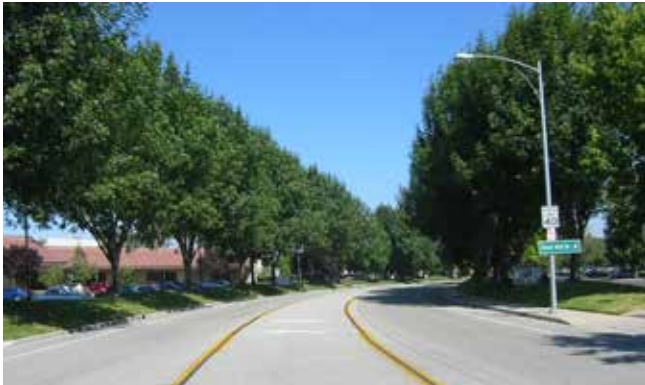
Single-story office development on McCandless Avenue that was constructed before 2008. (TASP)
