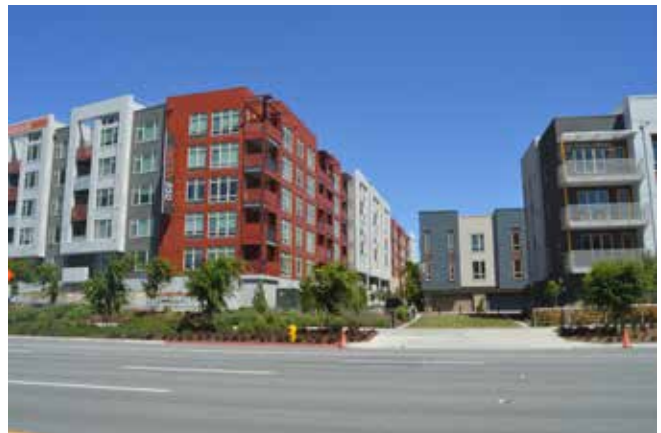
Capitol 650: New high density residential development at Montague and Great Mall Parkway.
