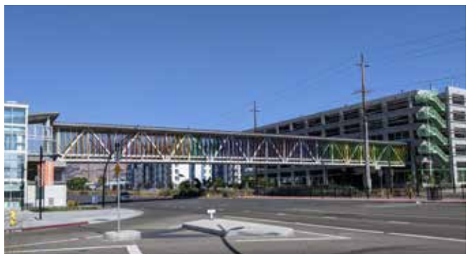
Public realm improvements near the Milpitas Transit Center include open spaces, streetscape improvements, and new pedestrian overhead bridges.
