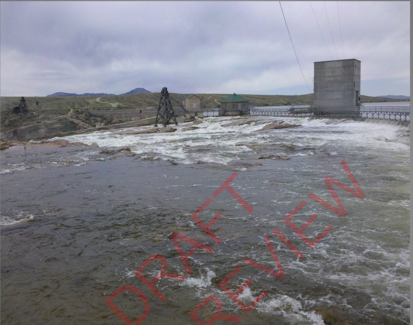
Photo: Pathfinder Dam Overflowing 2010
