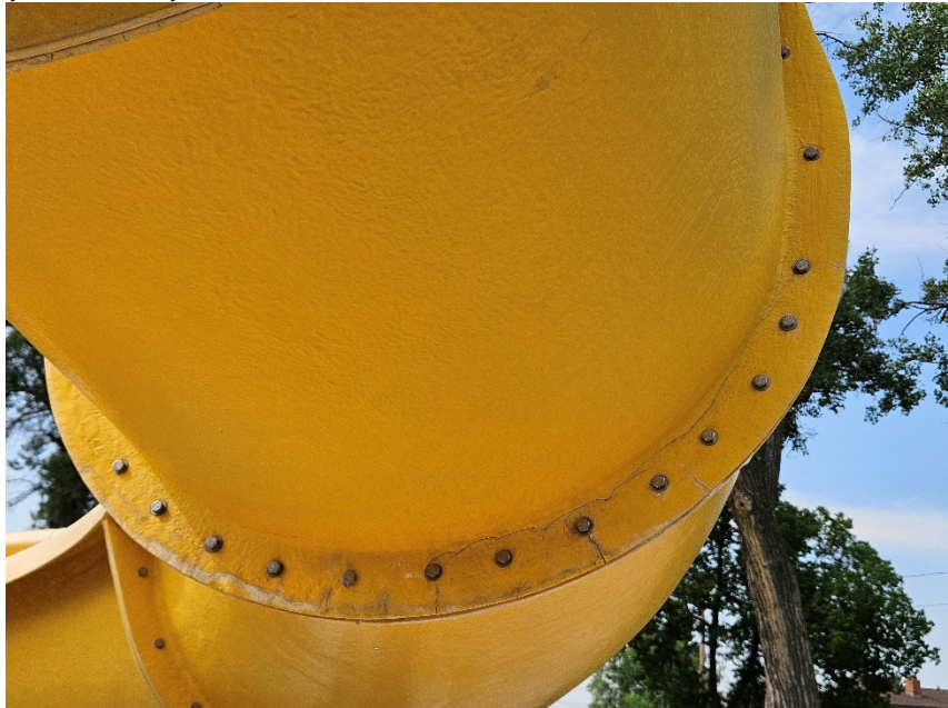
Figure 7: Cracked flange on waterslide.
