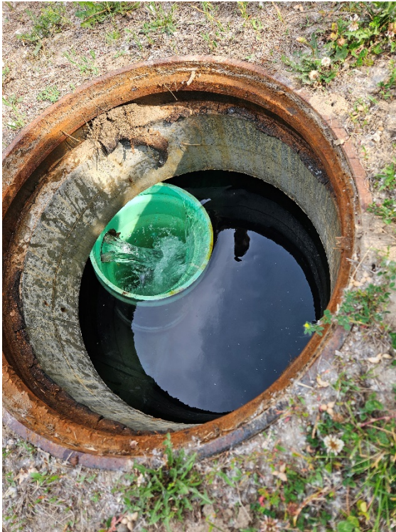
Figure 3: Strainer manhole full of water with standpipe.
