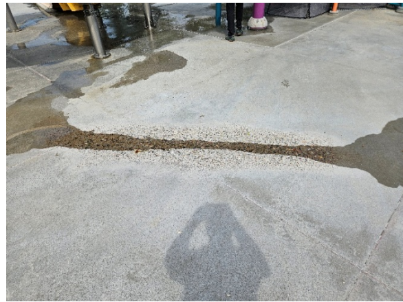
Figure 1: Concrete drainage grinding.
