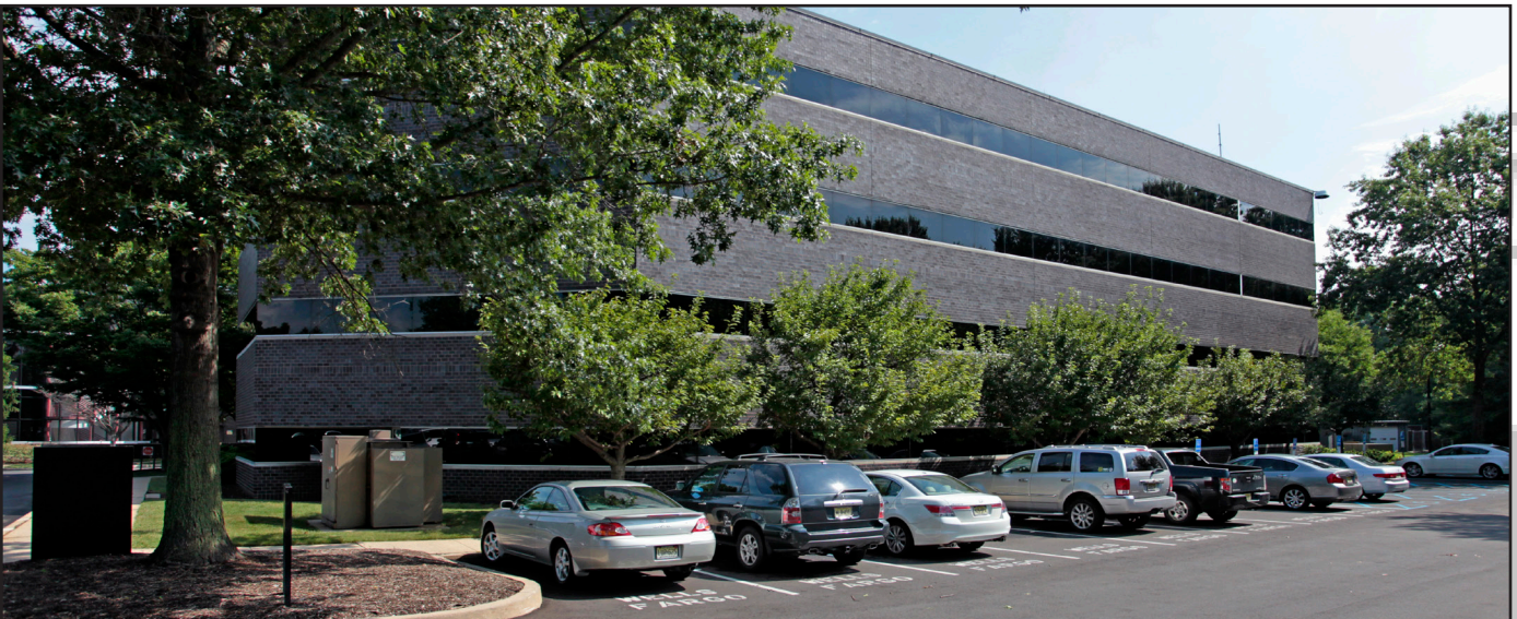
Image 3 - 7: Existing Office Buildings to Remain
