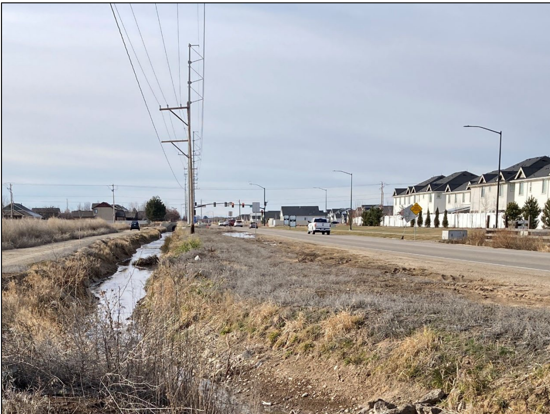
Figure 6. APE Overview showing Lemp Canal (10AA6408), View West, 1/18/2025.
