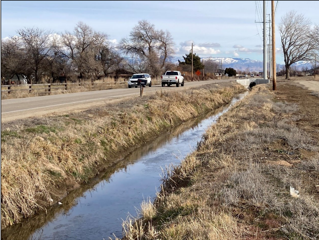
Figure 1. APE Overview showing Lemp Canal (10AA6408), View East, 1/18/2025.
