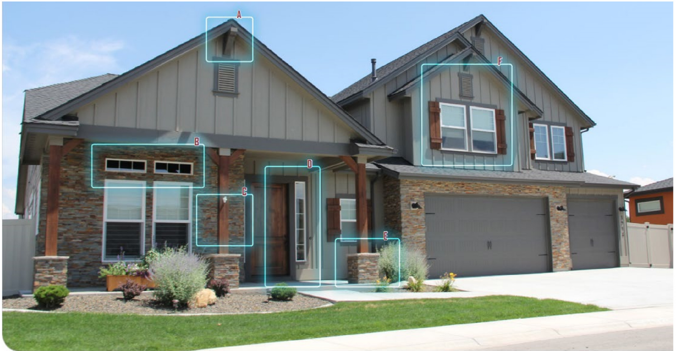
» This single family residential home has a number of added architectural elements including: {A} corbels to emphasize roof gables; {B} transom windows to create more interest; {C} stained wood columns and accents, to frame the entry and front of the house; {D} sidelights to emphasize the entry; {E} stone column bases with caps to anchor the building; and {F} shutters and trim around windows and vents to accent and transition materials.
