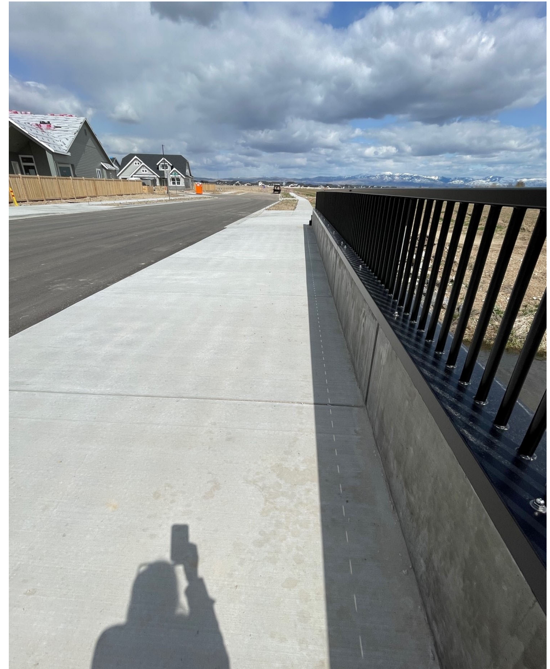
New bridge with pedestrian pathway component, Quartet Subdivision
