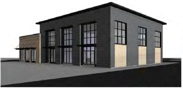
3 | SOUTH EAST CORNER
