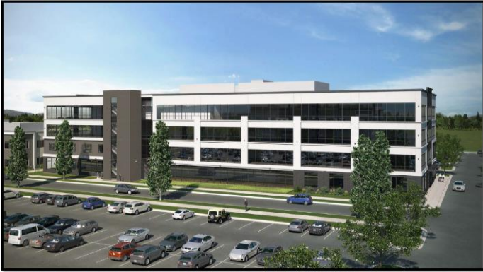
AMERIBEN PHASE II (under constr)
