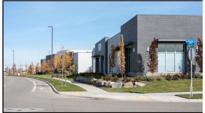
EXISTING SINGLE-STORY SHOPS
