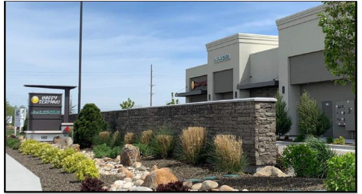
EXISTING RESTAURANT/SHOPS ( rear )
