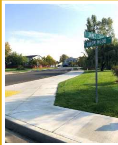
James Court Sidewalk Widening
